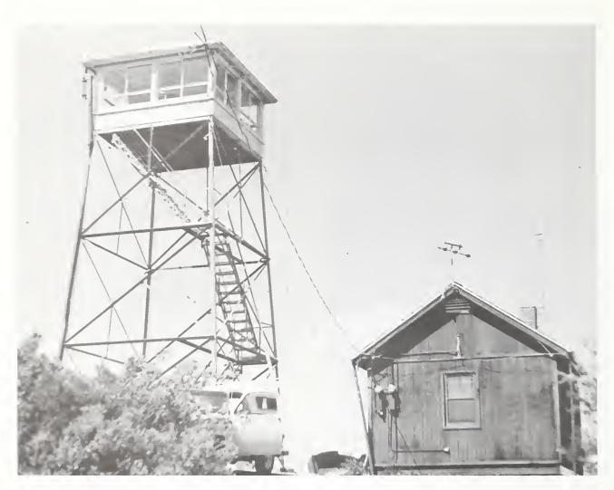
Figure 244. The Diamond Point lookout, an Aermotor MC-24, and cabin on the Tonto National Forest.
